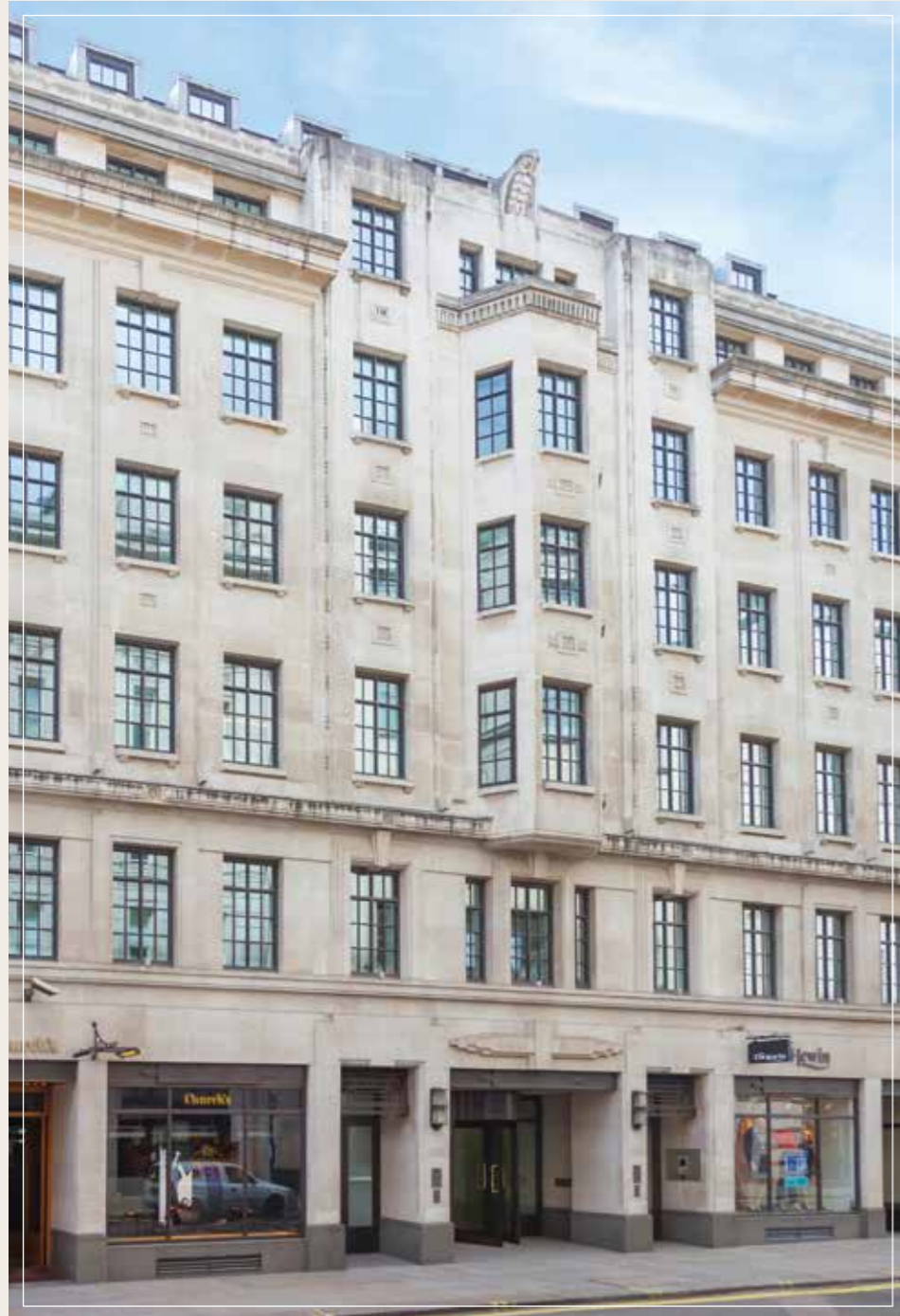
THIS LANDMARK CORNER OFFICE BUILDING IS SITUATED ON THE SOUTH SIDE OF JERMYN STREET IN THE HEART OF ST JAMES'S.
